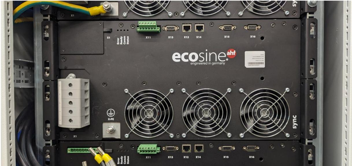
Figure 13-1 Example of a power module with all cables and fixation screws removed
